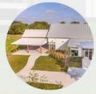
Pavilion Individual Room Rate
