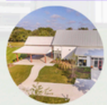
Pavilion Individual Room Rate
